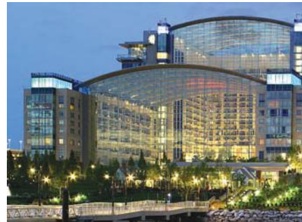
Installation of the 2,000 guest rooms at the Gaylord National Harbor Hotel
